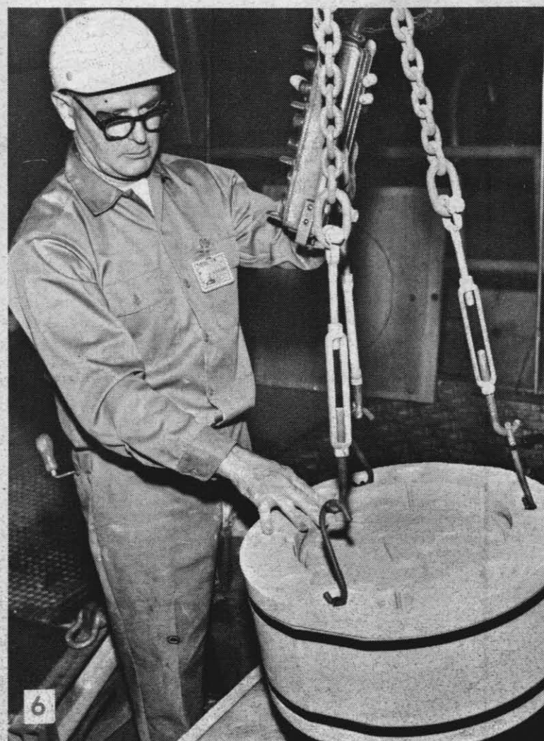
CORE ASSEMBLED TO THE MOLD
