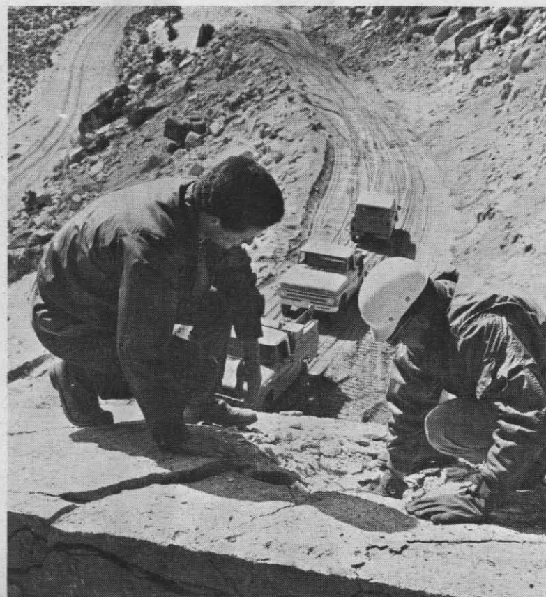
THE BIGGER THEY COME — The harder they fall. Cat driver Tony Serve (left) helps Lt. Dahlgren find where to put flaked TNT to split wounded boulder in half.
