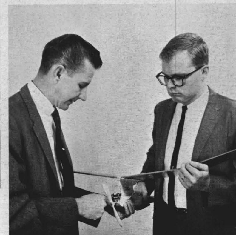
HIGH FLYER — Larry McMillin (left), builder and launcher of "UFO" which made unscheduled two-hour-plus flight to SNORT, cranks up .049 cubic inch engine with help of "co-pilot" John Wooldridge. McMillin has attached a "de-thermalized" device to tail for future flights in tricky desert air.
