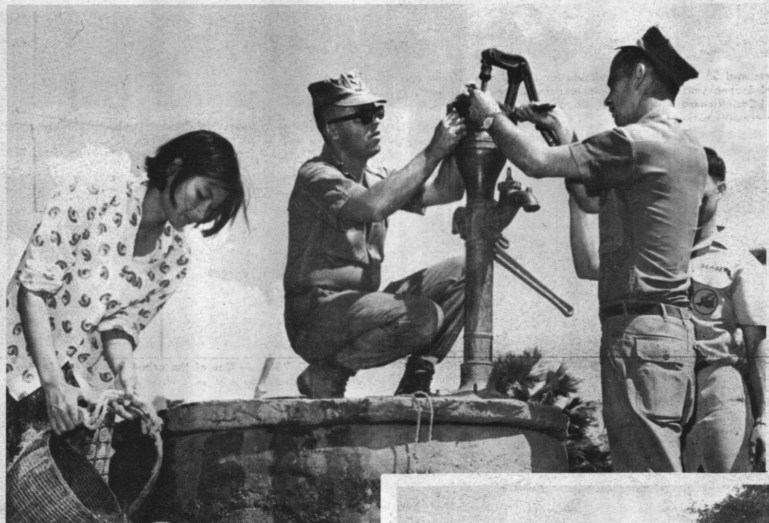
SEABEE TEAM — Corpsermen Daniel Buckley and Fred Nelson are engaged in repairing a village water pump after completion of their normal duties in Northern Thailand.
