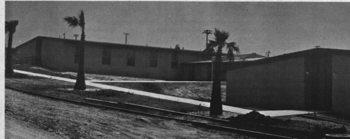
MOTEL TYPE, the BOQ has 20 rooms back to back. Exterior is light tan, brown trim.
