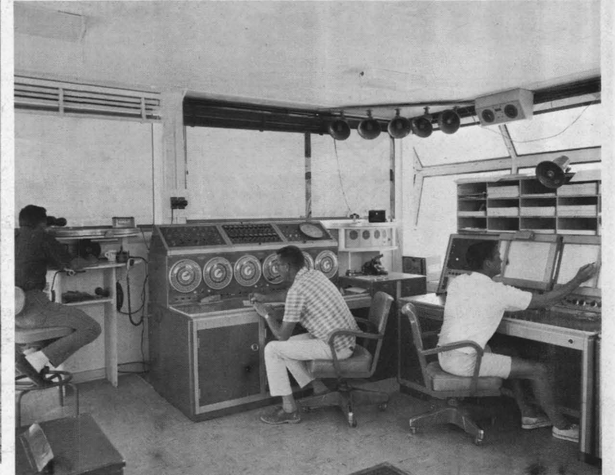
THE NERVE CENTER—This is an inside picture of the control tower at Charlie Range showing just a portion of the many intricate instruments that are used in conducting various tests. There are four different levels in the tower, each housing a vast assortment of these instruments. Note the picture at top center.
