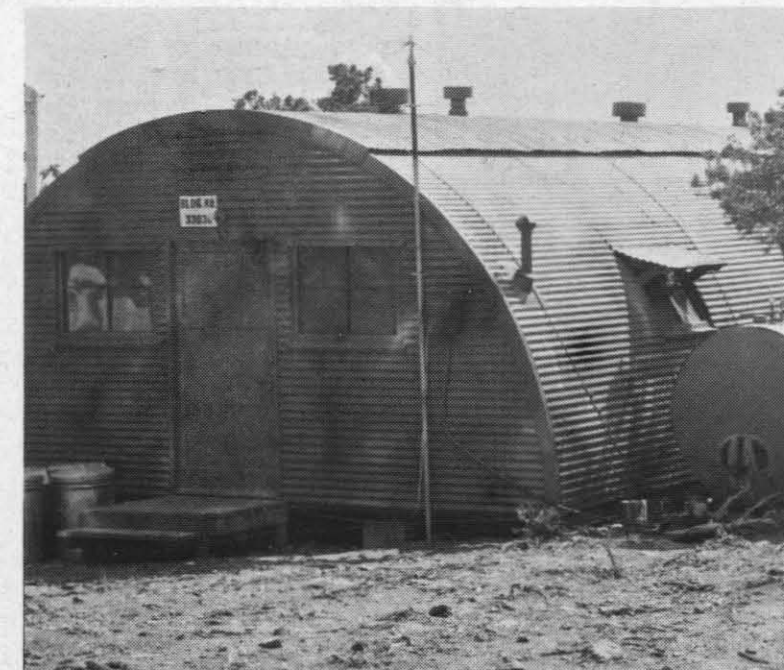
IT ISN'T MUCH BUT IT'S HOME — It may not look like much, but to those who have been here for a while it's a palace. This 20 x 40 foot Quonset replaced the two trailers that were formerly used for lodging.
