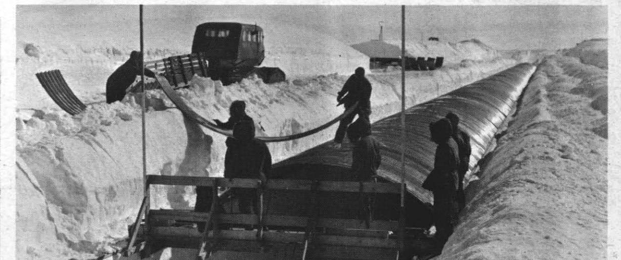
INSTALLING ARCHWAYS — These archways are placed over the tunnels above and then covered. It will then become the main passage, or main street, of the base.
