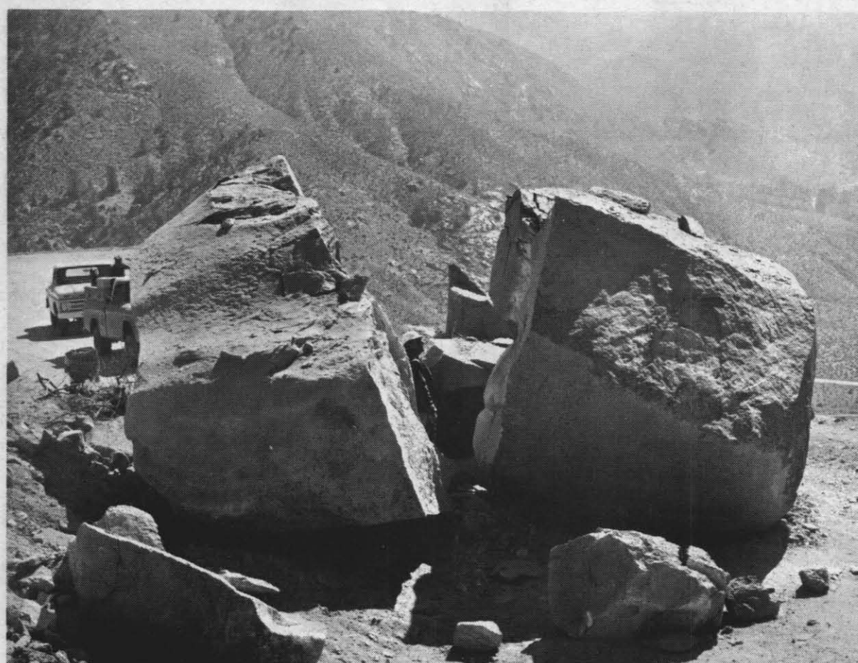
EFFECTS OF FIRST BLAST by two 40-lb. shaped charges is inspected by Lt. Dahlgren (center) after high-explosives split boulder
