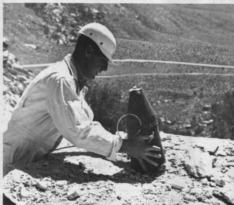
CHIEF WILSON of Explosive Ordnance Dept., places 15-lb. shaped charge on spot where it will do the most damage in second phase of blasting operation.
