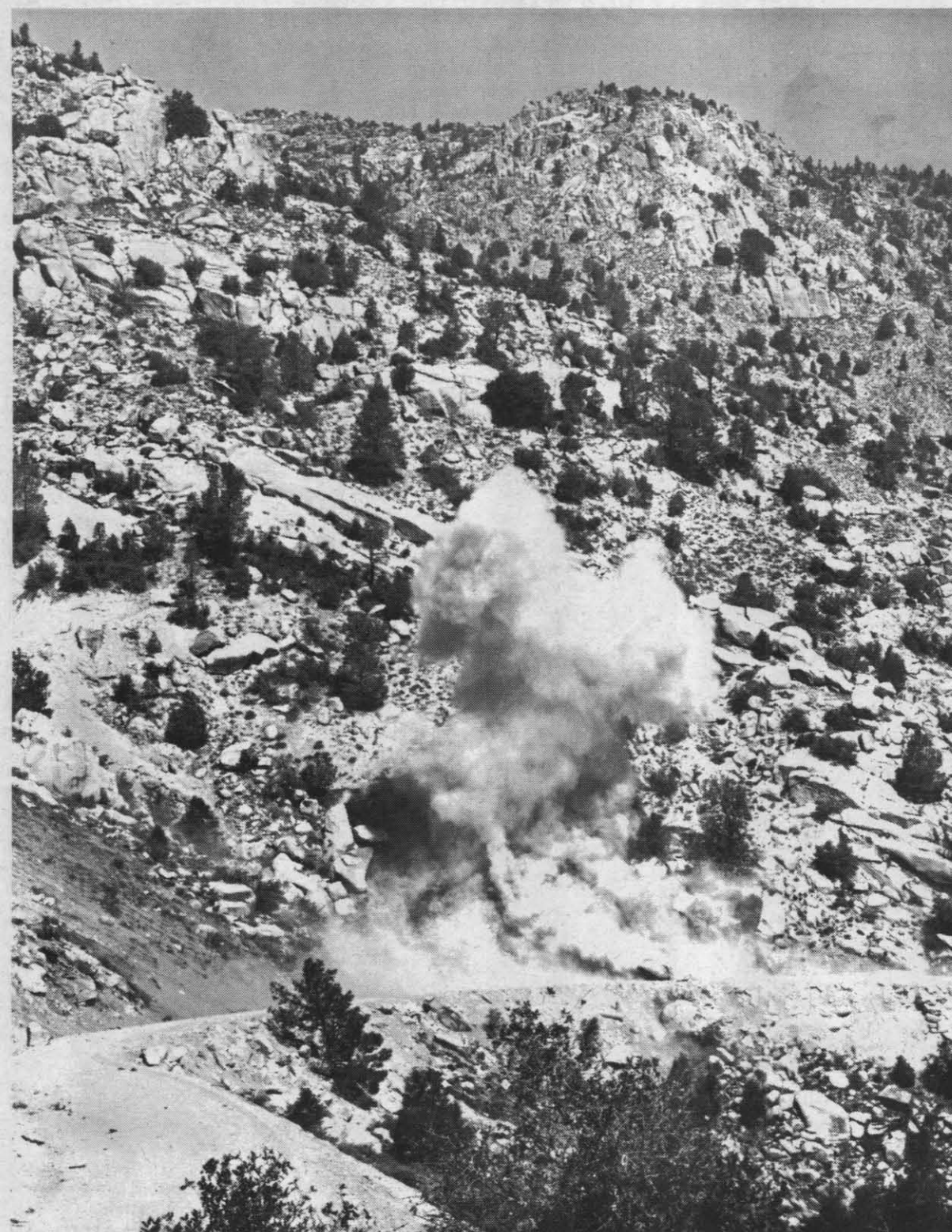
EARTH SHAKING BLAST of high-explosive shaped charges was recorded by photographer Willey from a quarter-mile distance. Explosion was the first of a series of three
