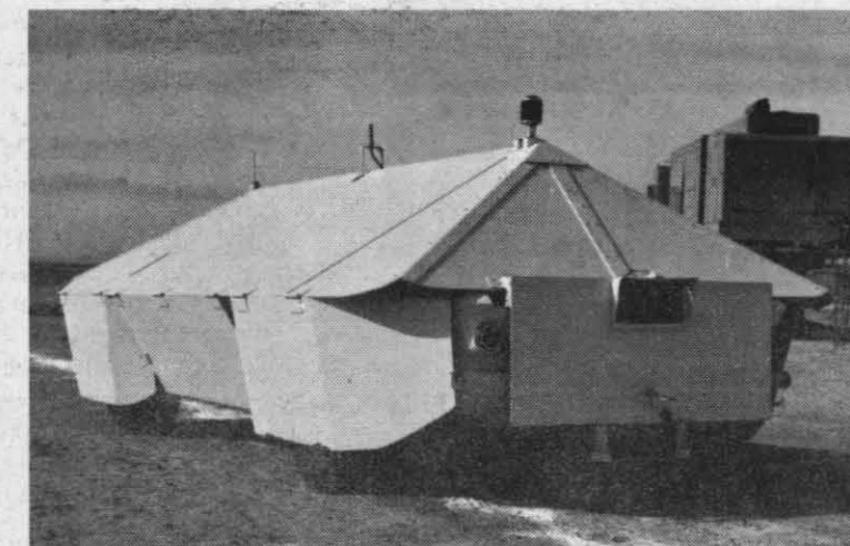
NOT A MOBILE PILLBOX —This is back end of remote-controlled Firebeetle. Concept could provide variety of moving targets for range commanders, among other applications. Television camera is mounted on front end.
