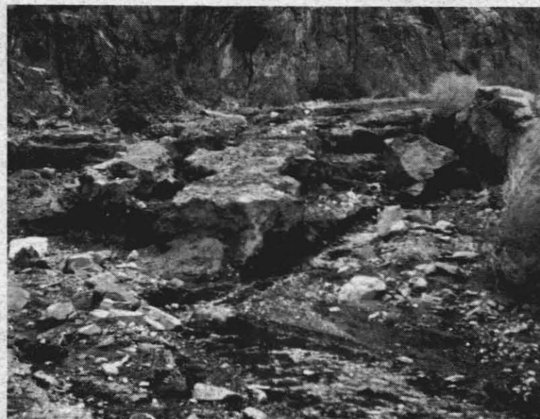
WASHOUT—Once passable road at Darwin Falls Canyon shows the work a heavy rain can do in just a short time. On the other hand, light or intermittent rain can smooth out a ragged roadbed.
