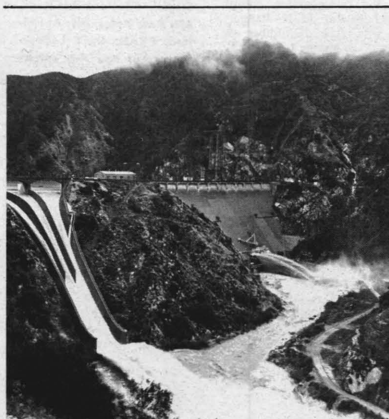
AND IT RAINED AND RAINED AND RAINED! —Pictorial evidence of the recent deluge is this photo taken below the Small Caliber Range at Morris Dam on Tuesday, November 23rd. The right side of the picture shows the bottom of the dam with water gushing through the needle valves at 3000 cubic feet per second. To the left of the picture shows the water pouring over the spillway at 7000 cubic feet per second. The needle valves are normally used to maintain lake level. The spillway comes into play at exceptionally high water level or flood stages.
