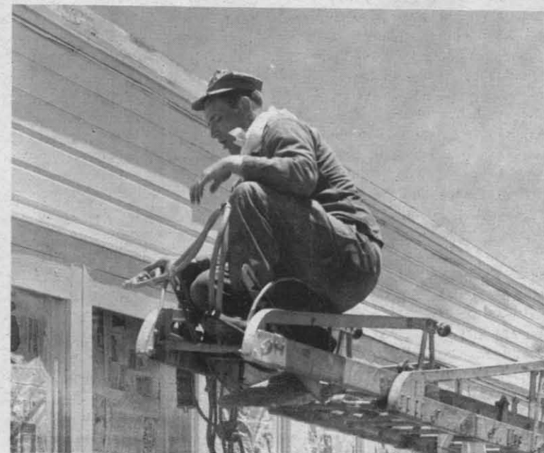
PAINTING EXCHANGE REC HALL at San Clemente Island is Marine reservist LCpl. Richard A. Jones, in civilian life an employee of the Georgia Pacific Plywood Co., at Eugene, Ore.
