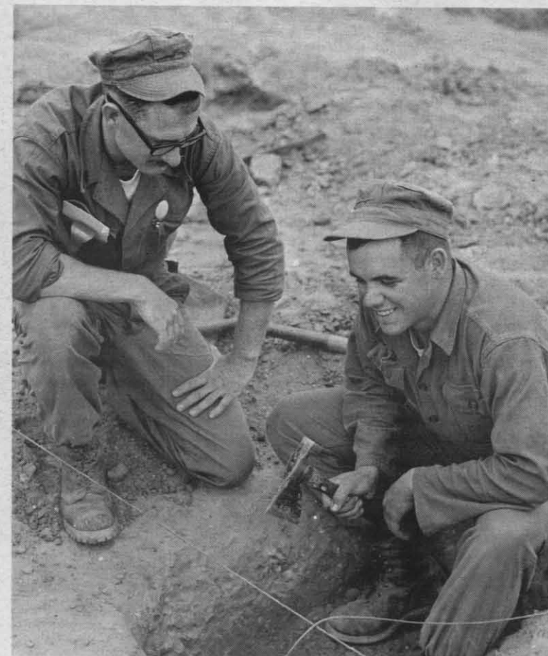
NEW WAITING ROOM ON SAN CLEMENTE ISLAND—Marine Reservists Sgt. Melvin W. Mitchell and Pvt. Lance J. Boyd, both from Portland, Ore., prepare a foundation for a new airfield waiting room on SCI during Portland, Oregon based Headquarters Company 5th Engineer Battalions' two-week summer training at Naval Amphibious Base, Coronado, Calif. Mitchel, a self-employed carpenter, is a part-time student at Portland Community and Portland State College. Boyd is a printer with Boyd Printing Company, Portland, Ore.
