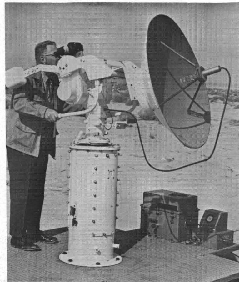
MANUAL TRACKING ANTENNA is operated by Roy E. Rockstrom of Code 40's Aeromechanics Div. It was first used for new VHF band tests in April, 1961. A second group of tests planned for this August, will use additional gear now in preparation by Code 30's Instrumentation Lab. A larger, trailer-mounted antenna is being converted from a Nike-Ajax tracking antenna to a "slave" unit for further testing this August.
