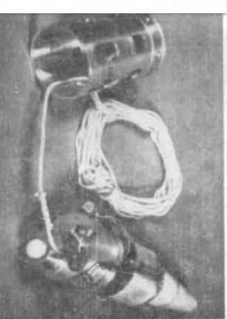
1250-POUND MISSILE was suspended in space using a stainless steel "air ball" tool to a tolerance of two microns. Here, Larry Ogan of Weapons Development Dept. activates infrared guidance system. "Air Ball" development is used to simulate "frictionless" altitude movement parallel "after burnout" conditions in space.
