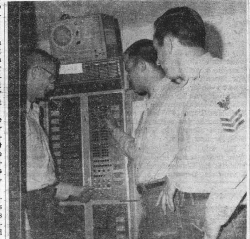
NAVY MEMBERS OF TEAM (from left) Frederick Krueger, DS1, Lawrence L. Hagadorn, FTMI, and James Stegall, FTMI, inspect digital computer complex that was conceived, designed, developed and tested at China Lake.
