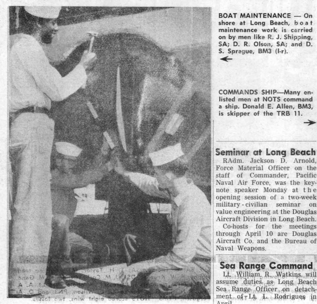
BOAT MAINTENANCE — On shore at Long Beach, boat maintenance work is carried on by men like R. J. Shipping, SA; D. R. Olson, SA; and D. S. Spreague, BM3 (I-r).
