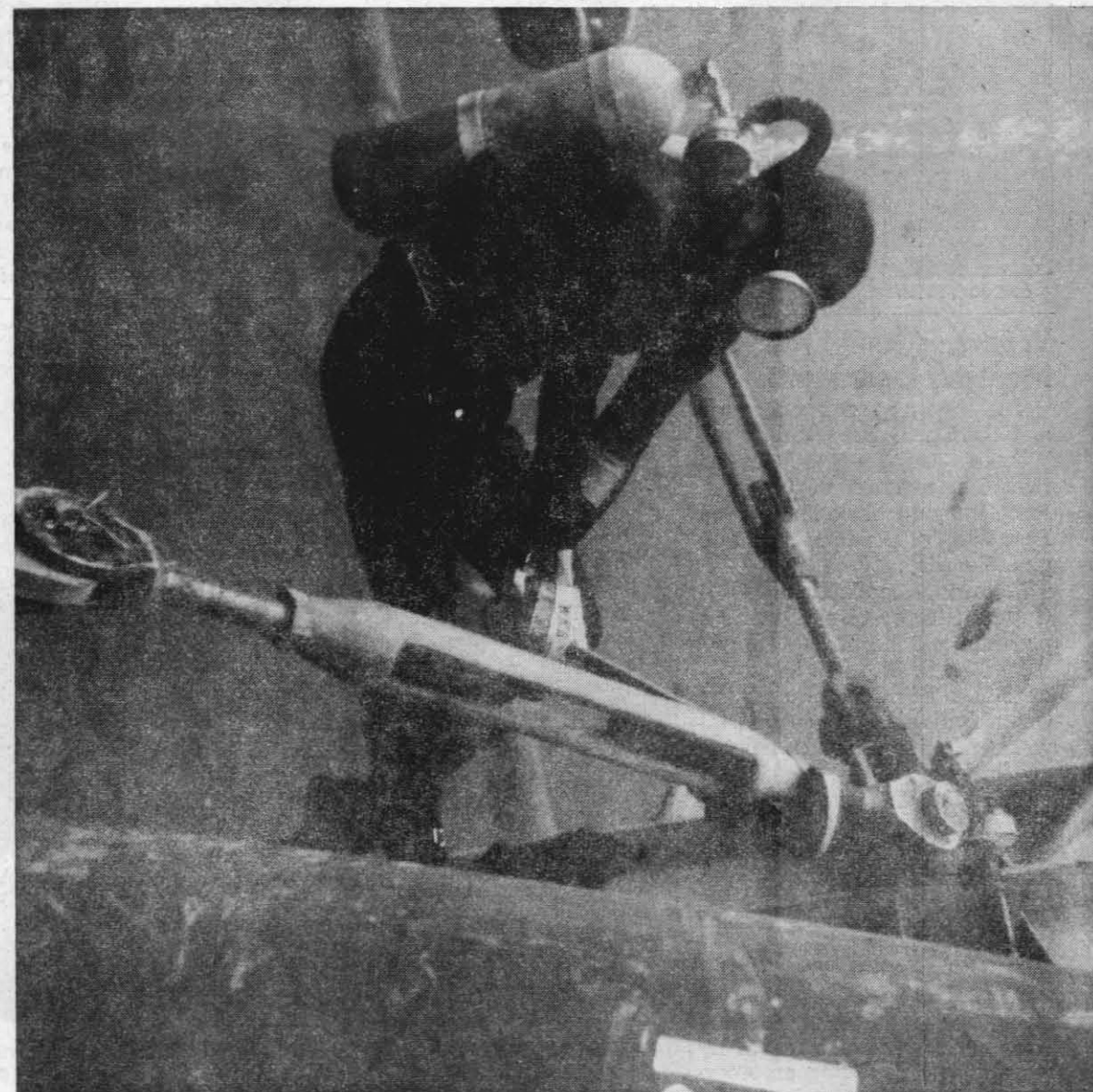
NAVY DIVER William R. Blewett uses big wrench to adjust translator guy wires.
