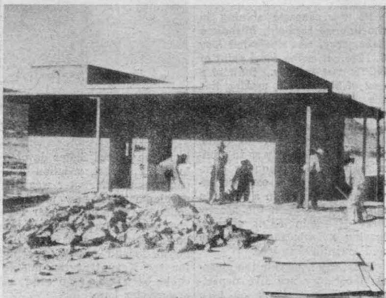
LABORERS level land around one of first buildings here.
