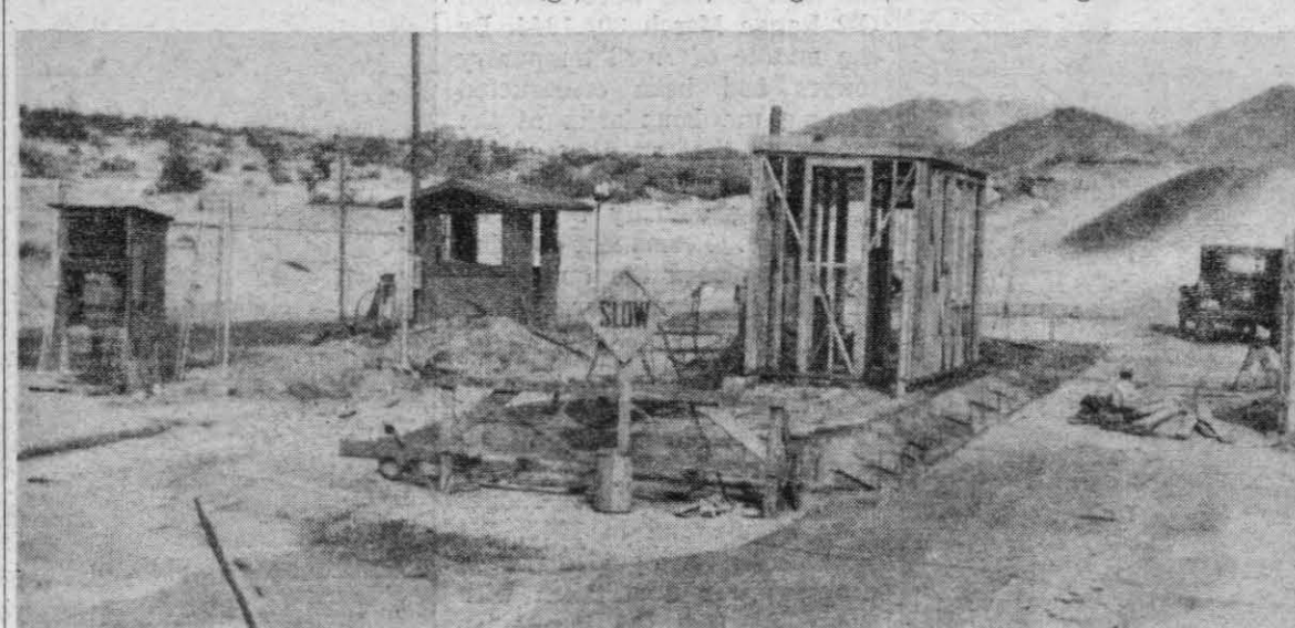
GUESS WHERE! — Picture was taken July 19, 1945. It's not the main gate sentry post, nor the one at the south entrance. But it is construction of guard gate leading to the Salt Wells Pilot Plant. Truly an historic shot. Road incline is the clue.
