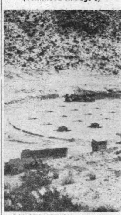
CONSTRUCTION of 1,500,000-gallon reservoir, June 15, 1944.
