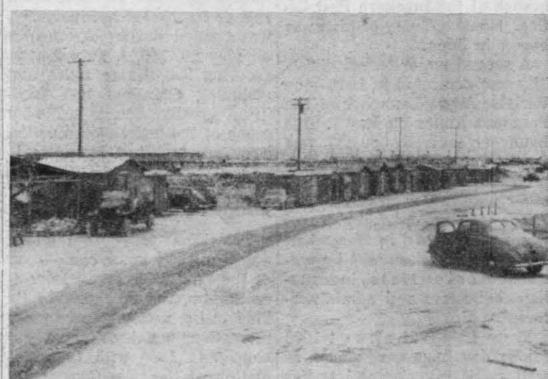
HURRIEDLY BUILT huts were "home" to construction crews.
