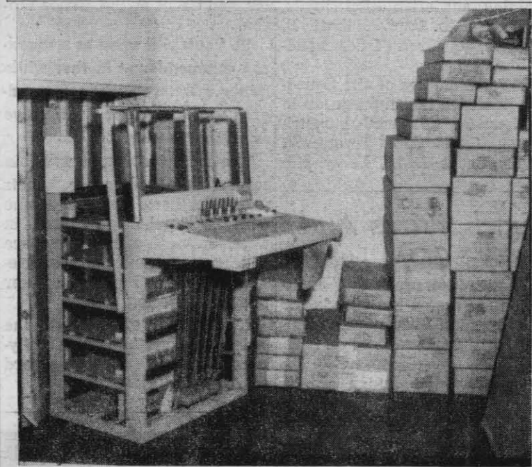
SPANKING NEW SWITCHBOARD will feature the latest thing in key pulse dialing. Installation is progressing rapidly.
