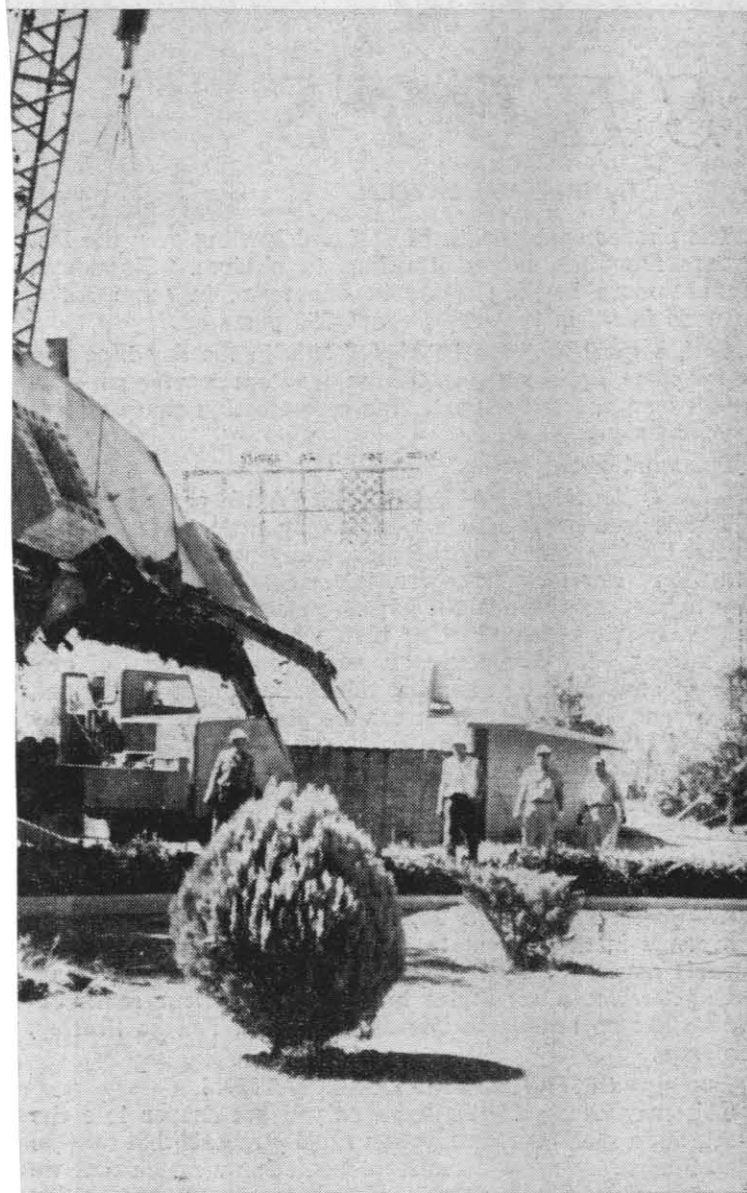
CPO Club dismantling total loss after blaze last October. Plans for a new club are well under way, but construction date is not yet determined.
