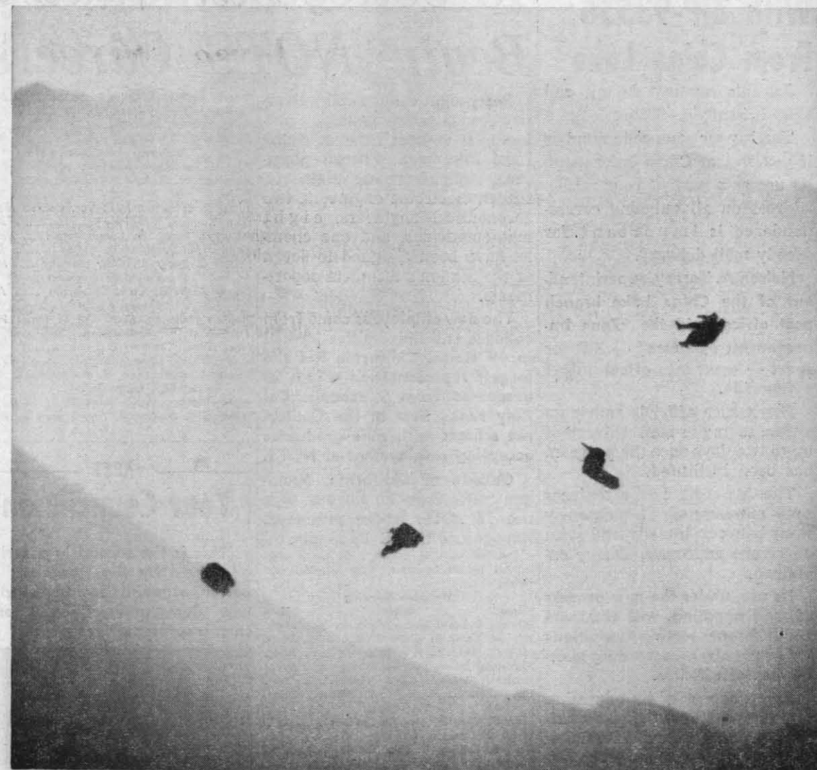
DUMMIES AND SEATS hurtle through the air, now at a safe distance from the "launch vehicle." That's the purpose, just in case of a malfunction at launch time.
