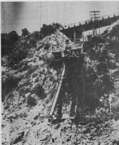
THE FIXED ANGLE LAUNCHER, during WW II, was the most valuable facility at the Morris Dam Test Range for simulating torpedo launchings with its 19 degree angle of launch.
