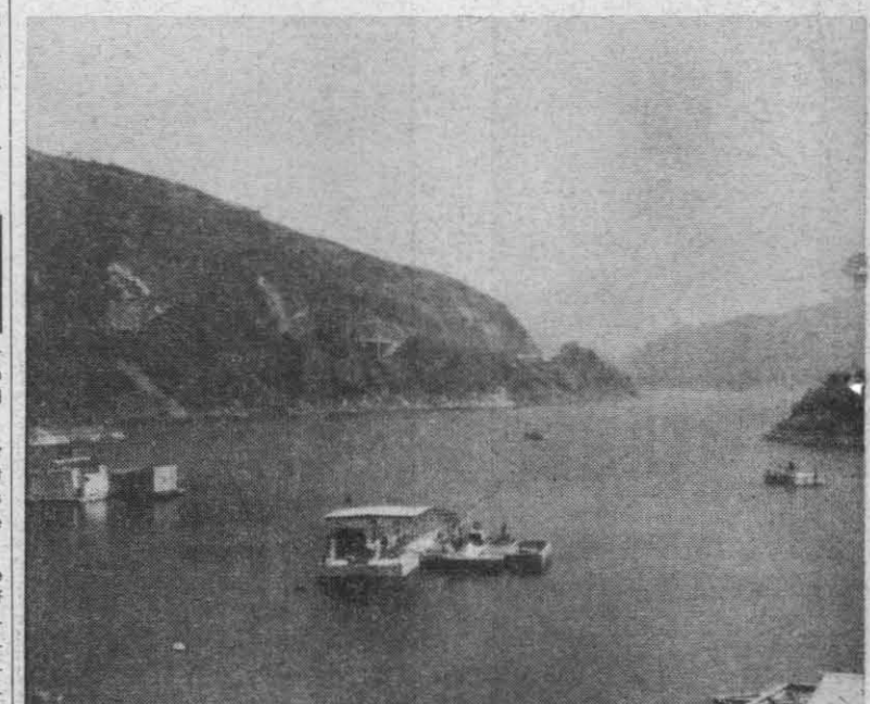
HILLSIDE VIEW—Looking north, the launching barge is shown in the foreground, and the transducer sonic barge to the left where sound equipment records pertinent data from test runs.
