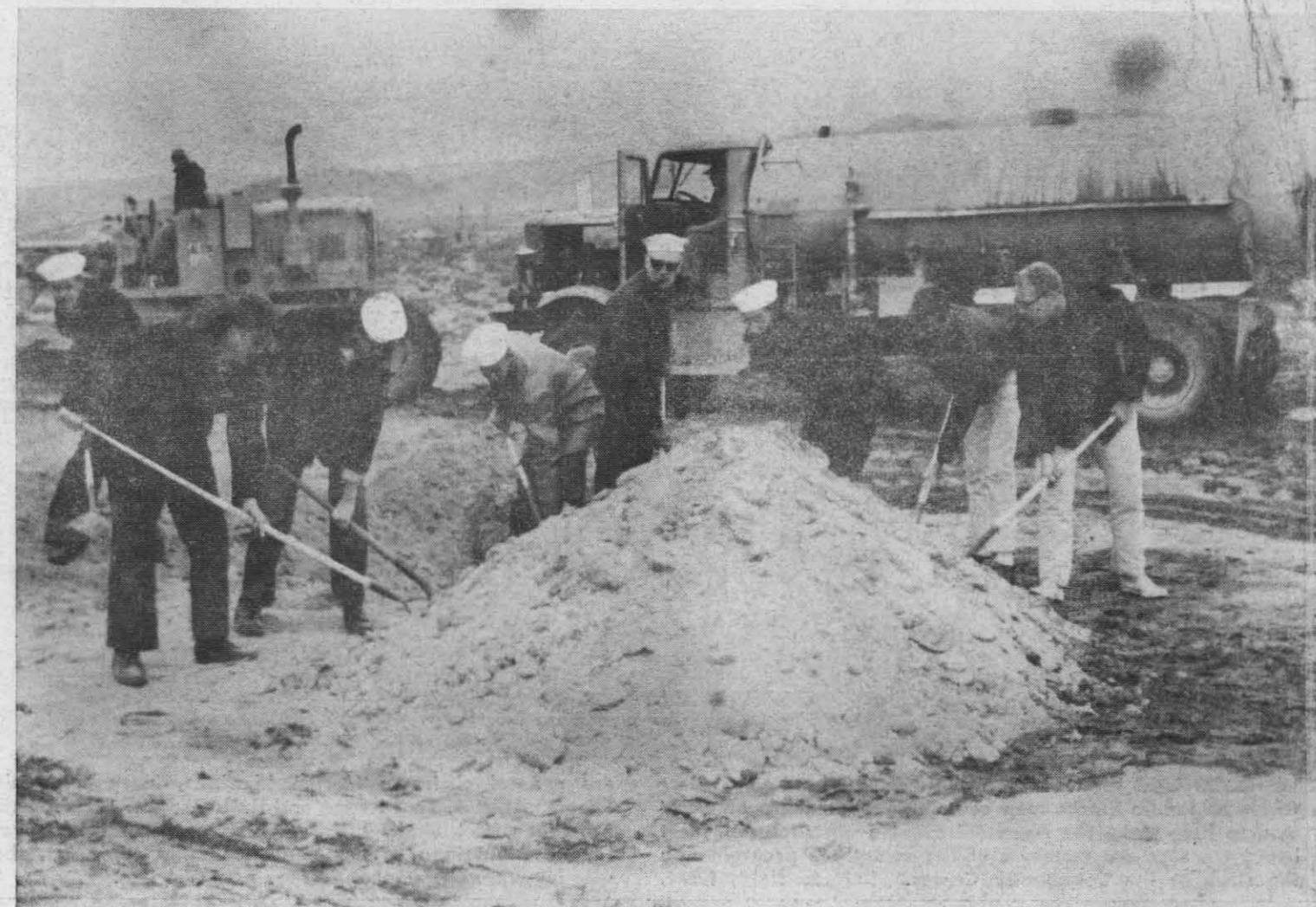
SEABEES ON THE JOB FOR LITTLE LEAGUE — Shovel brigade from the China Lake Construction Battalion turns to mound of dirt to level out the infield for the Ridgecrest-Inyokern Little League diamond at Downs and Dolphin Sts.
