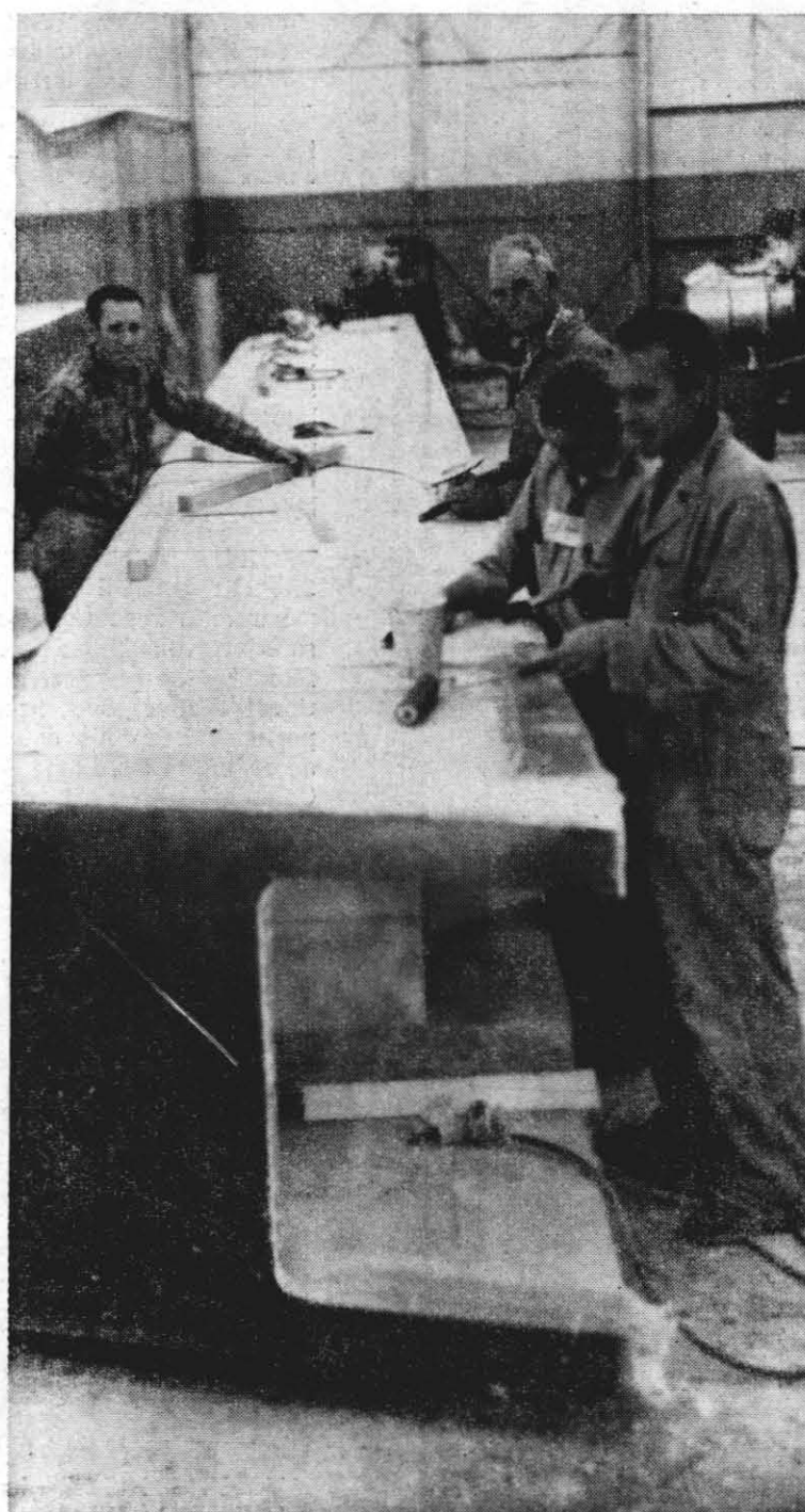
CATAMARAN PONTOON—Construction engineer Henry Hunnell (left) and Gordon Bredstrand, Ellsworth Smith, Bert Unger (front to rear) add the finishing touches to a 40' catamaran pontoon. Epoxy plastic makes rock-hard surface.
