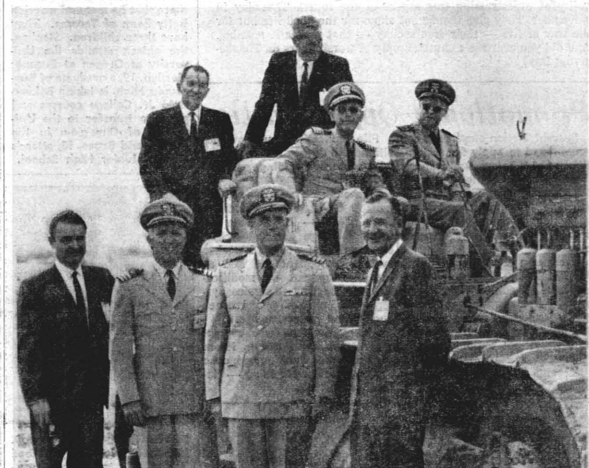
NEW INSTALLATION—Naval Air Facility Hough is Capt R. A. Davidson, Public Works Commanding Officer, Capt Jack W. Hough, takes the driver's seat in bulldozer to commemorate ground breaking for a Ryan Firebee jet target aircraft launcher to be installed by early next year. Seated alongside Capt
