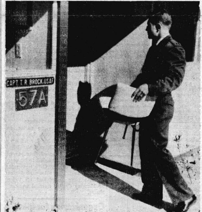
FIRST CAPEHART TENANT — Capt. Thomas R. Brock, USAF Liaison Officer attached to VX-5, lends a hand to settle his family in the first Capehart home move-in at 57-A Stroop Avenue on Monday, November 20. Nearly all of the completed 86 units at the site have been assigned in this first increment of 328 units adjoining Burroughs High School. The Capehart rental schedule will not be published in the Rocketeer, but the rates are available at the Housing Office.
