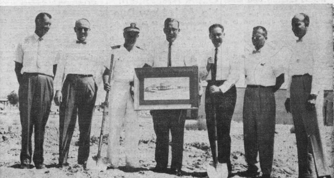
GROUND BREAKING—Station Commander Capt. Charles Blenman (3rd from left) is shown participating in ground breaking ceremonies Monday morning for the new California Interstate Telephone Co. building to be constructed on South China Lake Blvd. in Ridgecrest. Other participants (l-r) are W. T. Biggs, mgr. of the local telephone office; R. J. McCullough, American Potash and Chemical Corp. at Trona; Capt. Blenman; Johnnie Savage, Ridgecrest C of C president; Willard Wade, Interstate Telephone Co. president; Jack Bennington, prime contractor; and LeRoy Jackson, Head, Community Relations Office, NOTS. Estimated cost of the new facility is $169,000.
