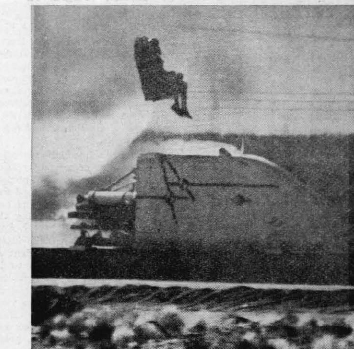
RAPEC — NOTS-developed Rocket Assisted Personnel Ejection Catapult seat ejects dummy to demonstrate how system will save lives of jet pilots faced with low-altitude crash emergencies. A static test firing of RAPEC will be conducted at SNORT today at 2:45 p.m.
