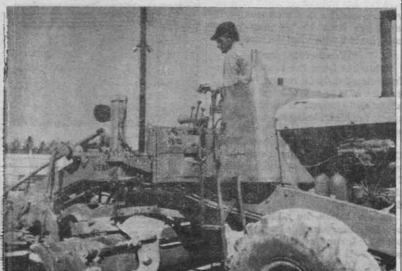
CB'S AT IT AGAIN—Louis Pipkin, one of the many volunteer workers from the Construction Battalion Division 11-2, operates a motor grader on Little League Diamond No. 1 in preparation for the season's official opening on Armed Forces Day. Restrooms will also be installed for the first time.
