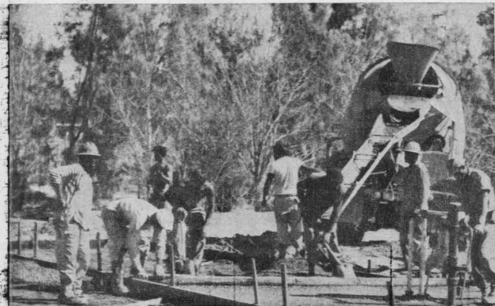
CAPEHART SLABS —Workmen are shown pouring a concrete slab for one of the 328 Capehart duplex units at Site "B" near the Burroughs High School. Approximately 110 slabs have been poured to date, according to Leon Berkovsky, project manager.
