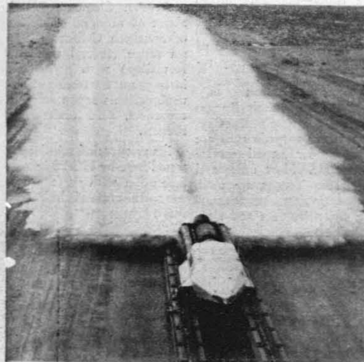
SNORT SLED—The artistically patterned spray following the moving sled on the SNORT Track will be seen today as the sled is slowed down by the water brake. A double bill will be featured at the Track today—a RAPEC demonstration at 1 p.m. and a High Speed Drag, nearing Mach 1, at 3:30 this afternoon.
