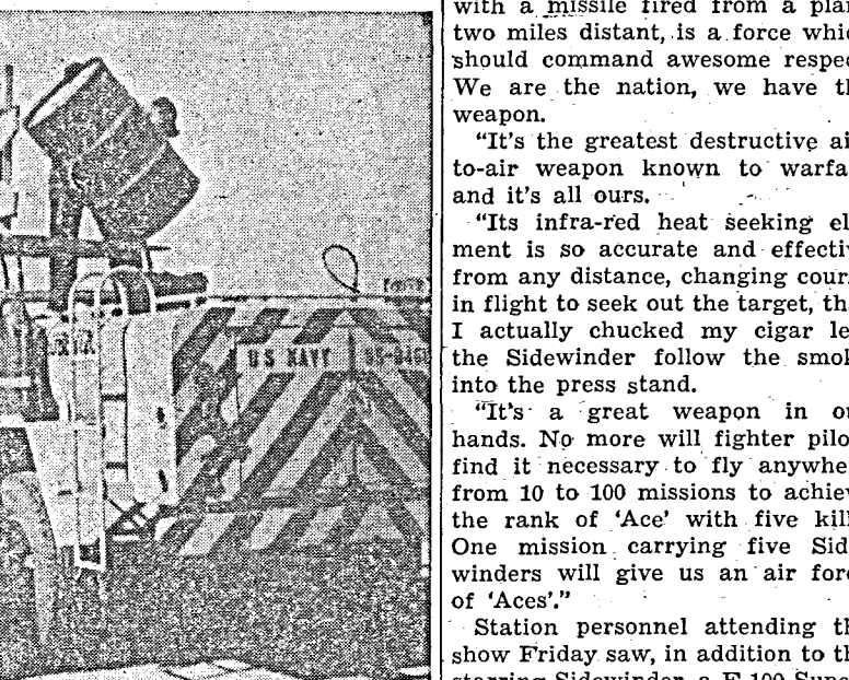
OLD METHOD —A fork lift hoists the oil drum in position over a funnel in the aviation lube refueler. Oil spilled over and drums could not be completely drained causing waste, oil contamination, and extensive cleanup work for the Public Works Department.
