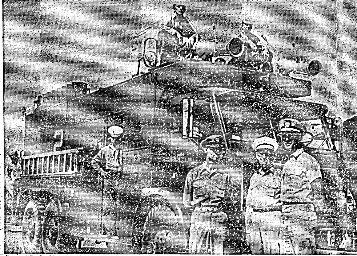
WHEELED GIANT—Part of the Station's fire fighting equipment are the MB-1 Crash and Rescue Trucks utilized at the Naval Air Facility. Featuring superior speed (64 mph), extreme mobility, an improved fire-fighting system and design and operational simplicity, the giant fire extinguishers can each cover burning aircraft with a 12,000-gallon blanket of foam within two minutes. N. E. Levy, AN, (left), and J. W. Stallman, AN, man the turrets atop the vehicle. R. G. Rascon, AN, (left), and D. H. Hudspeth (in doorway), fill two more of the five-man enlisted complement. R. A. Howell, Capt., Fire Dept., (left), and Roy D. Carter, driver, sit in the cab. Standing in front of the 17-ton vehicle (l. to r.) are: Cdr. A. O. Turner, NAF Operations Officer, Fire Chief A. C. Wright and Cdr. E. H. Gunther, USN, NAF Fire Marshall. Powered by a 320 hp Continental engine, the vehicle maneuvers well in rough terrain. Fire Apparatus to Parade through Housing Area Saturday, October 11. To promote fire consciousness, one MB-1 Crash-Rescue truck will be entered in the Desert Empire Fair Parade tomorrow morning. On October 11, fire fighting equipment will tour the housing area.
