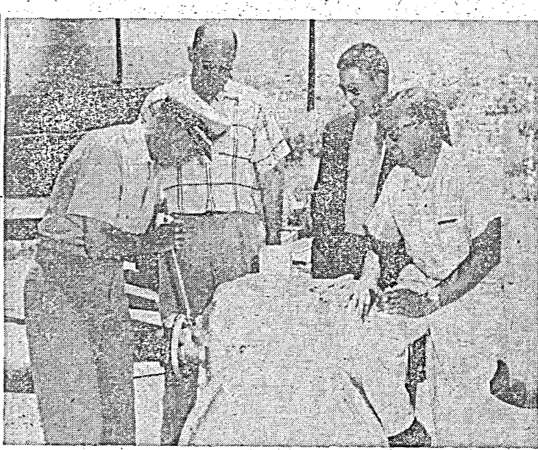
NATURAL GAS WILL FLOW—Public Works Officer Capt. G. H. Carrithers makes the final adjustment on the master meter which controls the flow of natural gas through the Station lines. Observing (l. to r.) are: Maurice Lipp, Head Eng. Div.; PW; E. C. Shaw, Master Mechanic, PW; and Bob Grimes, Pacific Gas & Electric Construction Superintendent.
