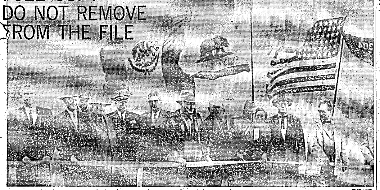
HIGHWAY 395 DEDICATION —Acting as representatives of the Station, Captain F. A. Chenault, Station Executive Officer and the Rev. John L. Reid Jr., NOTS Community Church pastor, (fifth and sixth from left) observe Paul Hubbard, Ridgecrest publisher, cut the ribbon which marked the formal opening of the newly-realigned section of U.S. Highway 395 at Inyokern last Friday. Independent Photo
