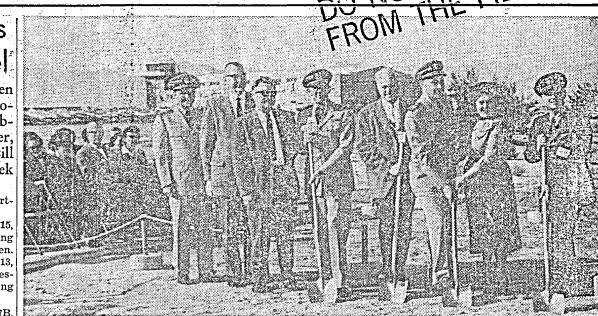
GROUND BROKEN —Groundbreaking ceremonies launched the new $3,500,000 hangar construction at NAF on December 30. It marked a new era of expansion for the Station. Participants in the ceremony (l. to r.) are: Capt. R. A. Beveridge, VX-5; Dr. A. G. Hoyem, Head, Aircraft Projects Div.; Hack Wilson, associate technical director; Capt. G. H. Carrithers, resident officer-in-charge of construction; George Bronaugh, Diversified Builders, Inc.; Capt. G. J. Anderson, NAF; Assemblywoman Dorothy Donahoe, 38th (l. to r.); and Capt. W. W. Hollister, Station Commander. More than 100 persons witnessed the ceremony.
