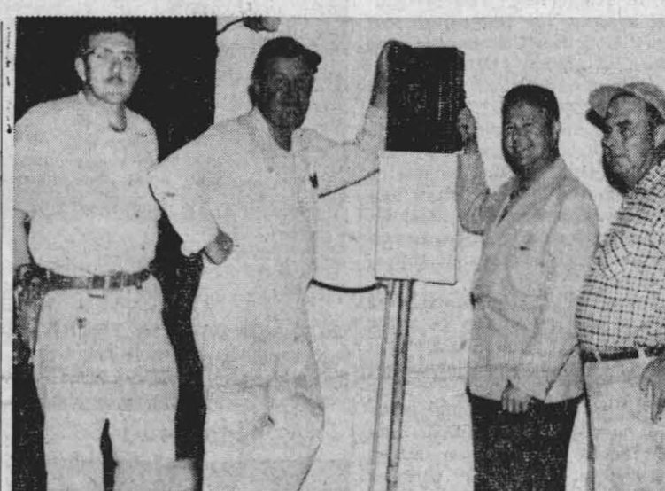
PROJECT POWER LINE FINALE—Another stride in the direction of progress is completed when the switch is pulled and electricity replaces fuel oil at Laurel mountain TV booster station.
