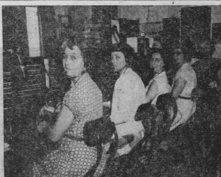
SWITCHBOARD OPERATORS—Seated at the board (l. to r.) are: Libby Toth, Georgia Smith, Evelyn Coit, and Hilda Walbert. Standing in the rear is Peggy Nichols, assistant chief operator.
