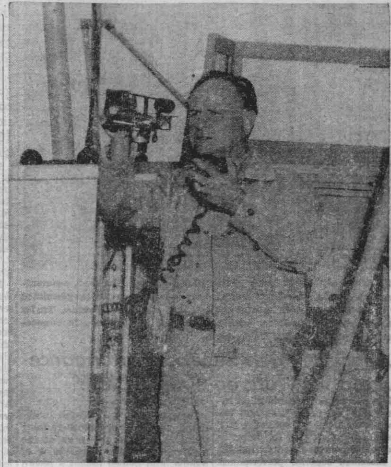
LONG BEACH TEST CONDUCTOR—In this picture, Fred Lux, ordnance experimental test mechanic, is using the stadiometer to station a target boat at a specified distance during a project at sea.
