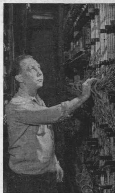
EXAMINING the cross connector banks at the Station telephone exchange is Herbert P. Hood, apprentice telephoneman.
