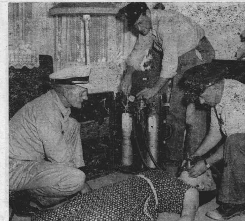
A DEMONSTRATION in the use of the portable resuscitator carried by the fire and rescue truck is given by Fire Chief K. T. Faust, left, William LaCombe, operating the oxygen supply bottles, and John Nevey, shown demonstrating the use of the resuscitator's mask. "Victim" for the demonstration was Mrs. K. T. Faust, who offered to assist the men during the training session.
