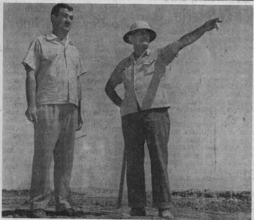
LAYOUT of the new nine-hole golf course is being explained to Paul Somerson by L. C. Smith, construction superintendent. If the present construction schedule is maintained it is anticipated that local golf enthusiasts will be playing on the course about next June 1.
